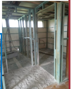
Sprinkler system install left, framework for new toilets right
